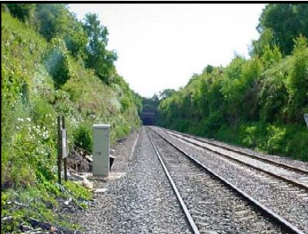
The view toward the Welsh portal from the location used by RAYNET operators during Exercise “Brunel”. A fair distance to get the radio signals into the tunnel before exiting the other end!
